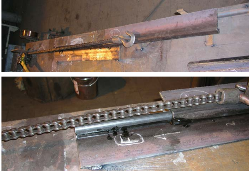
Figure 8: Insertion of the panels (LARSEN Interlock)
