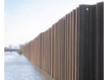
▶ London Avenue Canal, New Orleans
