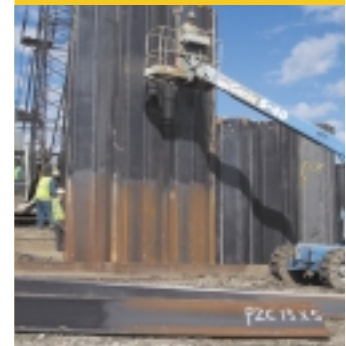
▶ IHNC Levee Rebuilding, New Orleans
