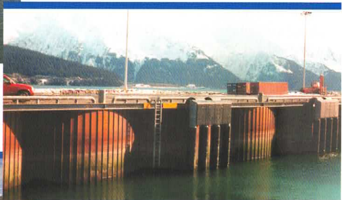
Open Cell Dock, Seward, Alaska
