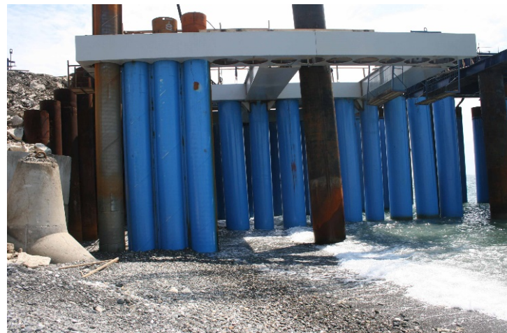
O-Pile template in marine environment
