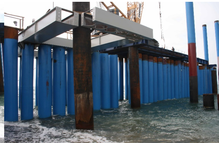
Another angle of O-Pile template in marine environment
