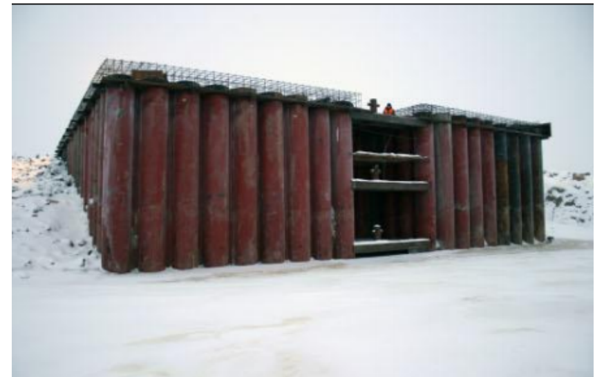
Example of O-Pile structure in extreme weather elements
