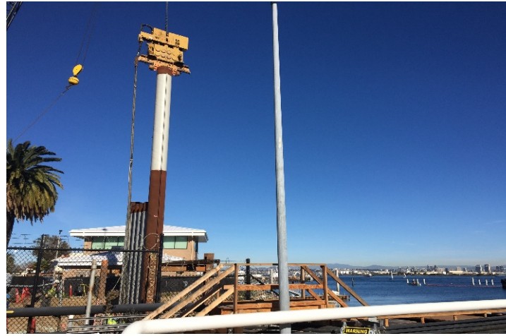
Impact hammer driving an O-Pile
