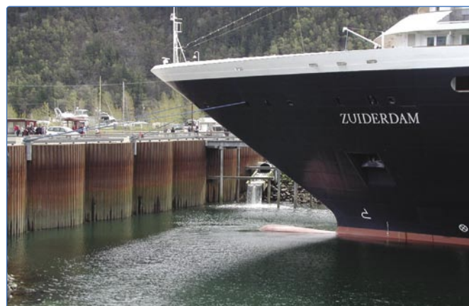
Figure 5. Broadway Dock Expansion.
